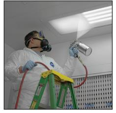
6. Spray 945 Crystal Clear on lights and windows. No masking required. 945 is transparent over white.
