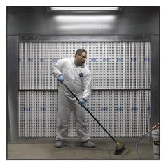
1. Clean contaminants from walls, lights, and floors. Apply prep coats if necessary.
