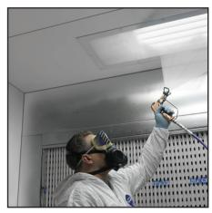
4. Spray Carbicote White to completely cover booth ceiling, lights and windows. No masking required.
